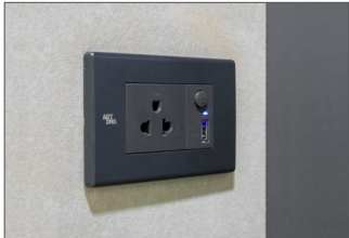
Electrical Outlet and USB Charger
